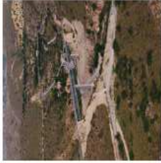
NUDO CARRETERAS - VÍAS TREN ROAD JUNCTION - RAILROAD TRACKS 38°27'36,4"N 0°20'40,9"W
