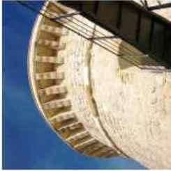
TORRE RENACENTISTA RENAISSANCE TOWER 38°25'57,9"N 0°23'02,1"W
